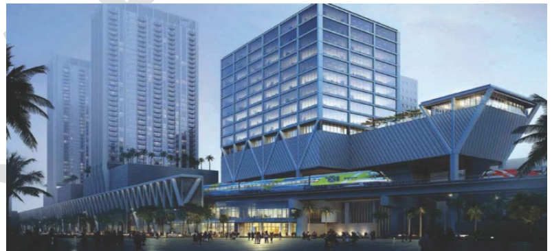
Figure 25. Miami Central Station, the southern terminus of the SMART Plan Northeast Corridor.
